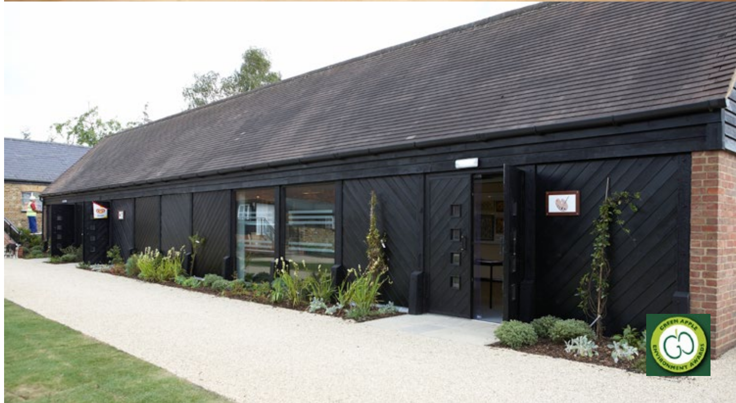
Top Image: Restored timber frame of the C13th Grade II* Great Barn.
