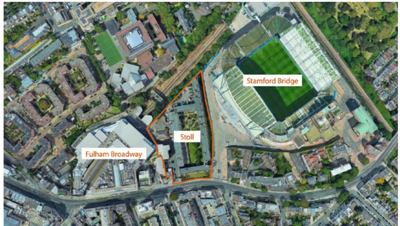
Above Image: Aerial view outlining the current Stoll property. Main Image: Illustration of the proposed redevelopment of Stoll Mansions.
