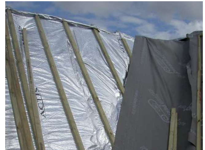
Images Bottom and Top Right: Enhanced insulation to roofs can be achieved by re-slating using modern multi-foil insulation materials.
